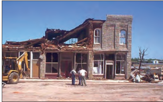
Surveying the damage in Stockton, Mo.
